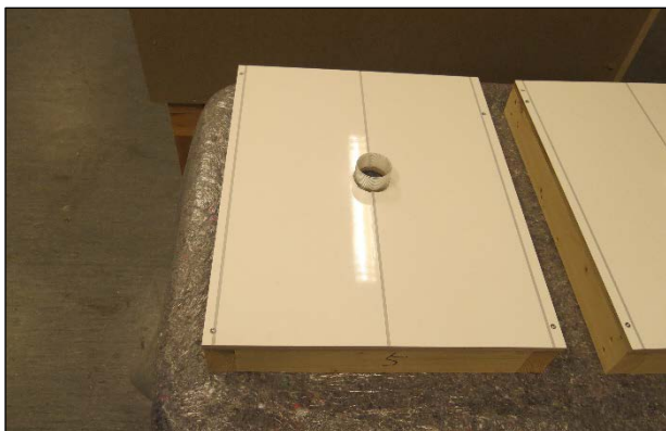
Fig. 5.1.1: Inserting of Roth QuickBox in Fibo bathroom wall panel.
